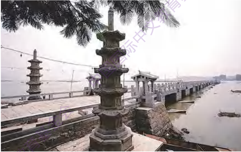
泉州洛阳桥 Quanzhou Luoyang Bridge
